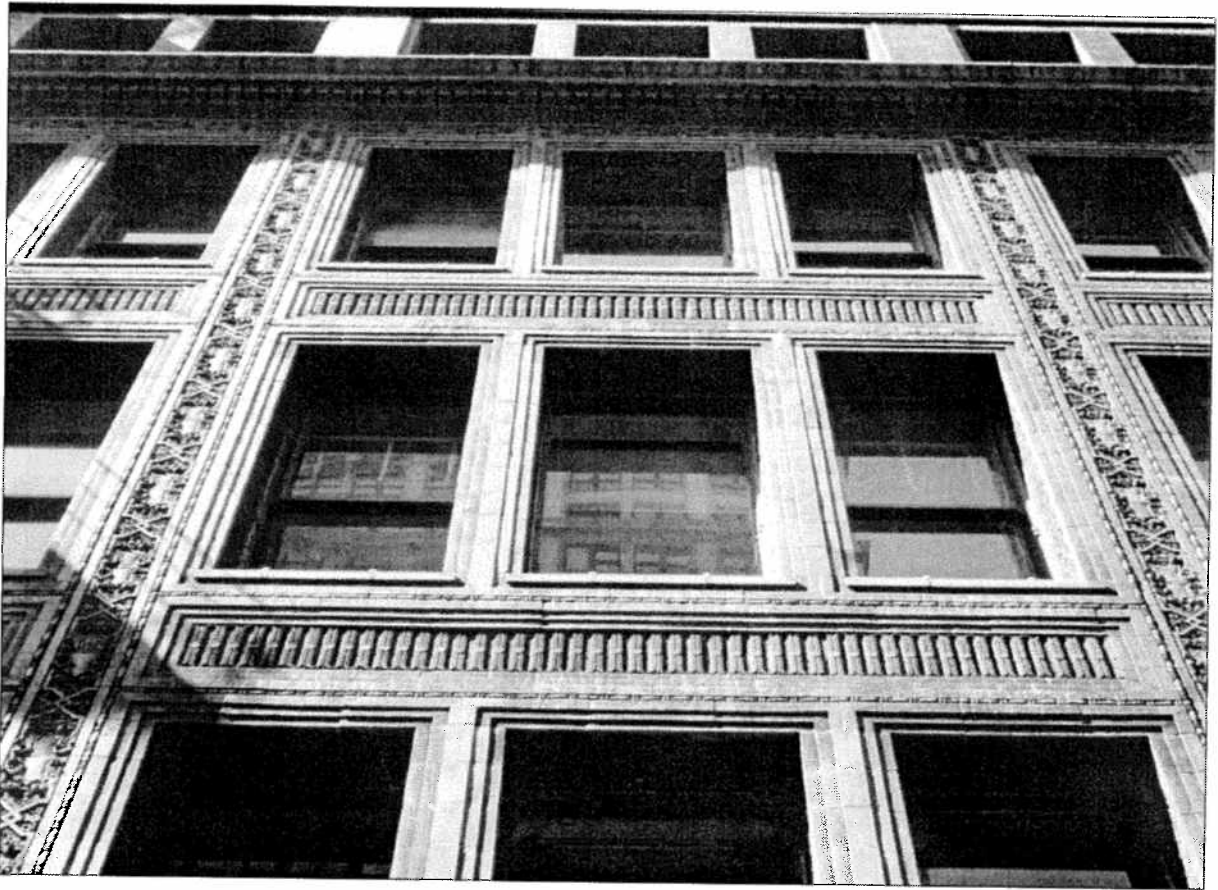
The high-relief terra-cotta ornament on the Heyworth Building creates strong patterns of light and shadow, giving the building an appealing human scale.
